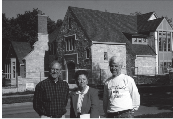
Chris Mitchell, Mary Wade, and Dave Lutz in May 2001 during the construction of the Wade Center.
